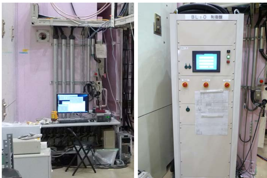
Fig. 3 The former controllers and drivers for two slits and a goniometer (left), and the newly integrated one (right).
