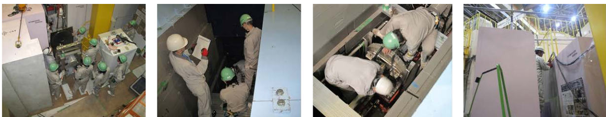
Figure 3. Damage investigation of chopper systems, beam-transport, shielding by technicians.
