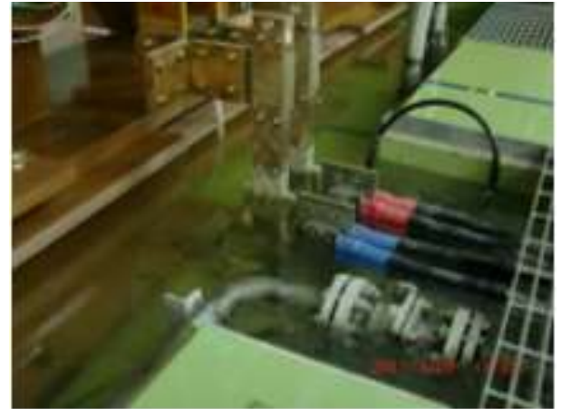
Submerged cables and connectors
