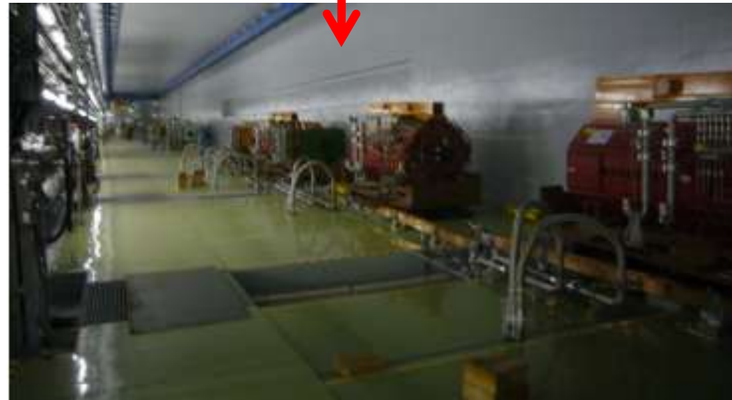
Realignment of switchyard magnets is in progress.
