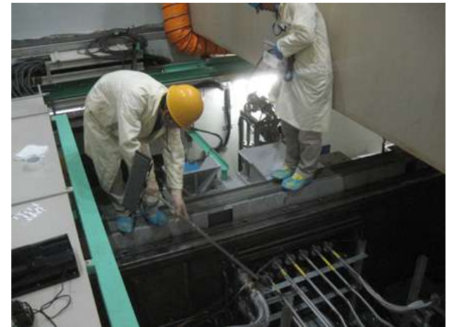
Measuring radiation level with opening a cover of the station 23
