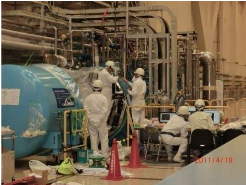
Inspection of Expansion Turbine
