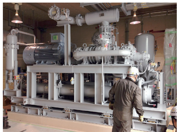
Fig. 3. New helium compressor for the MLF muon D-Line magnet system.
