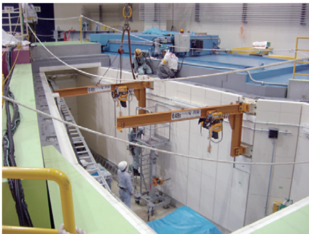
Fig. 8. Construction of the external building
