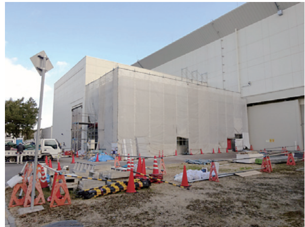
Fig. 7. Construction of BL22 (RADEN)
