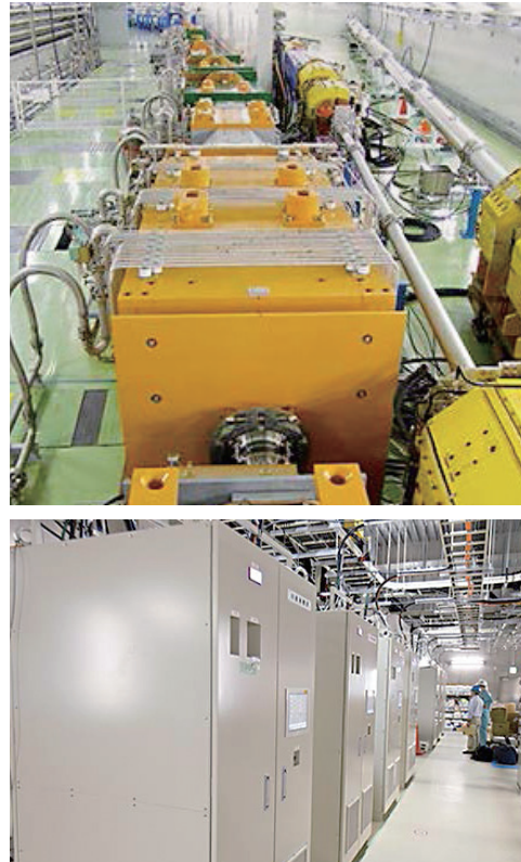
Fig. 4. (top) Normal conducting magnets of the primary proton beam line, and (bottom) their new power supplies.
