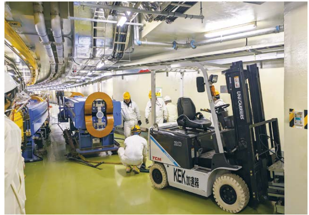
Fig. 17. Replacement work of the main bending magnet
