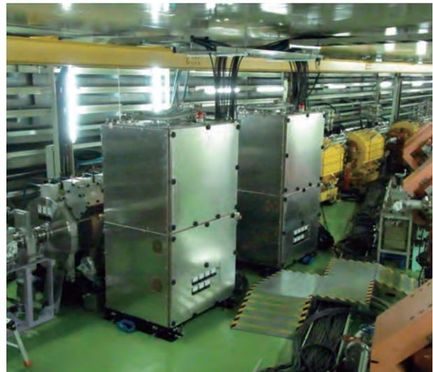
**Fig. 16.** Two RF cavities and power amplifiers installed in the insertion A.
