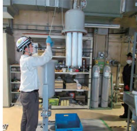
Fig. 4. Exchange work of the second oil separation filter.
