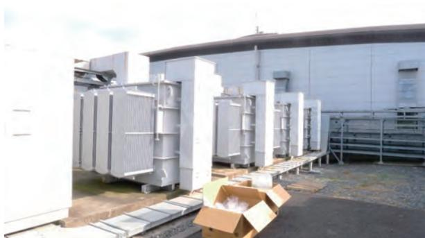
**Fig. 14.** The transformer - rectifier assemblies of the RF system.
